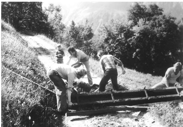
Strassenbau in Brün 1975
